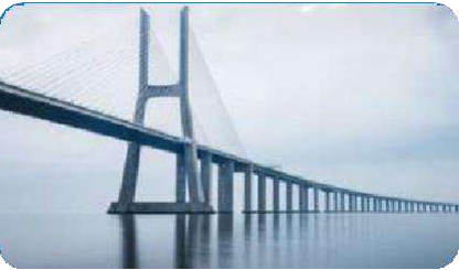
Bridge Piers Monitoring
